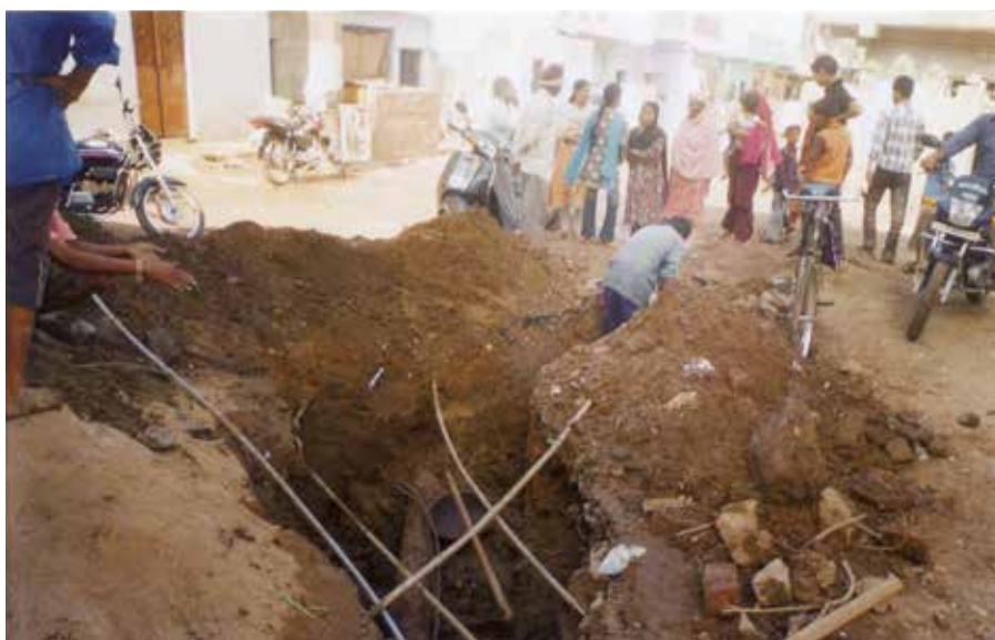
Drainage work undertaken by the municipal corporation through community pressure
