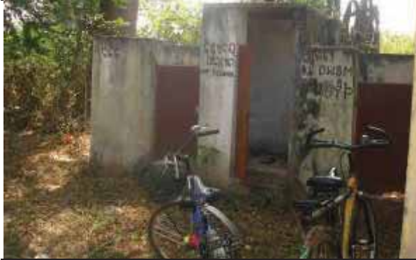
Non-functional toilets a common feature of all schools visited
