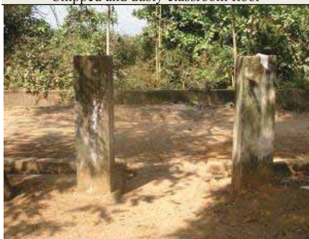
Several schools visited had no boundary wall, playground or gates
