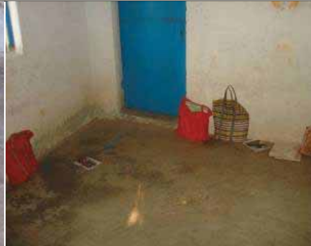
Bathroom built attached to the classroom
